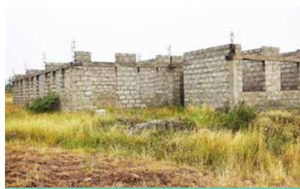
Administration blocks at Moroto remand home that is still under construction
