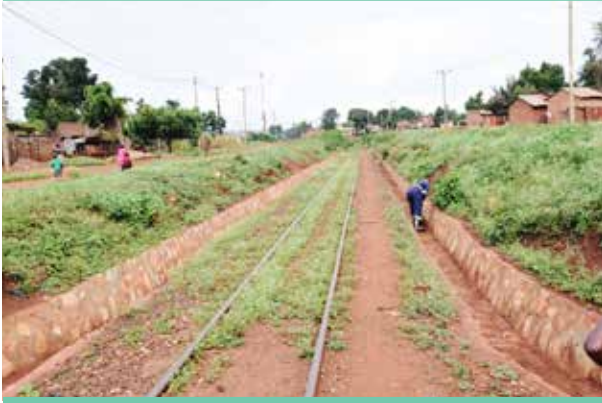
Railway rehabilitation at Magamaga and Budumbuli
