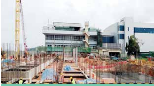
Expansion works at Entebbe Airport: Passenger Terminal
