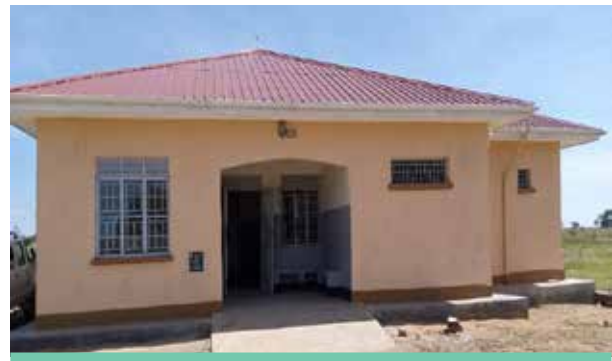
Newly constructed Apeitolim Police Station in Napak district
