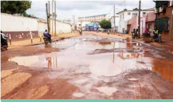
A road in industrial area - Kampala
