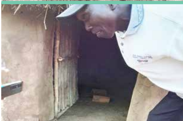
UHRC officials inspect a newly constructed and well-maintained pit latrine at Okuda Police Post
