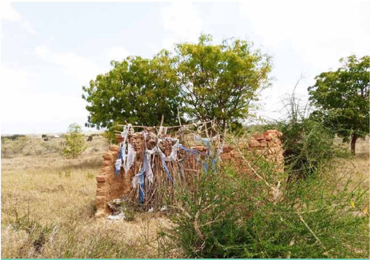
Bathing facility at Lorengedwat police station in Nabilatuk district.
